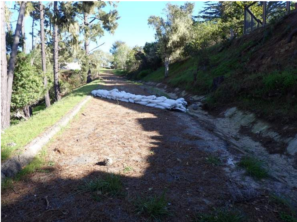
Photo 2. View of sandbags used to direct road runoff into the swale as part of the interim erosion control efforts.
