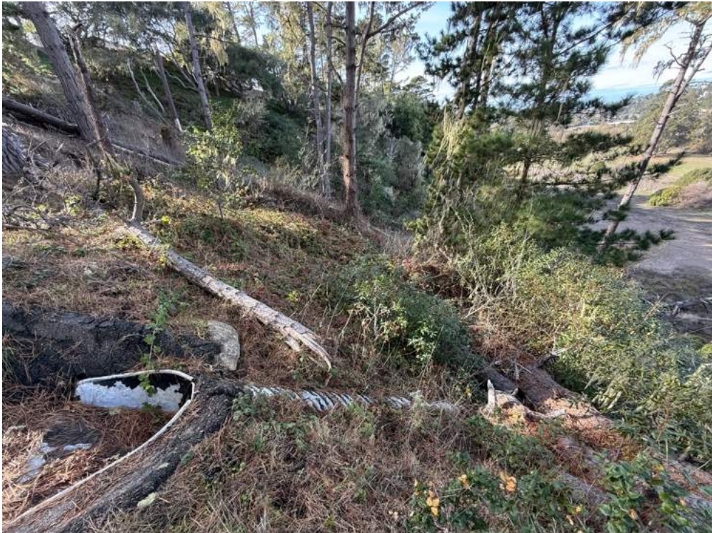
Photo 14. View of the storm drain pipe that carries surface runoff down to the lower slope and floodplain. The new, upsized storm drain pipe would be laid on the ground adjacent to this pipe, and vegetation impacts minimized.
