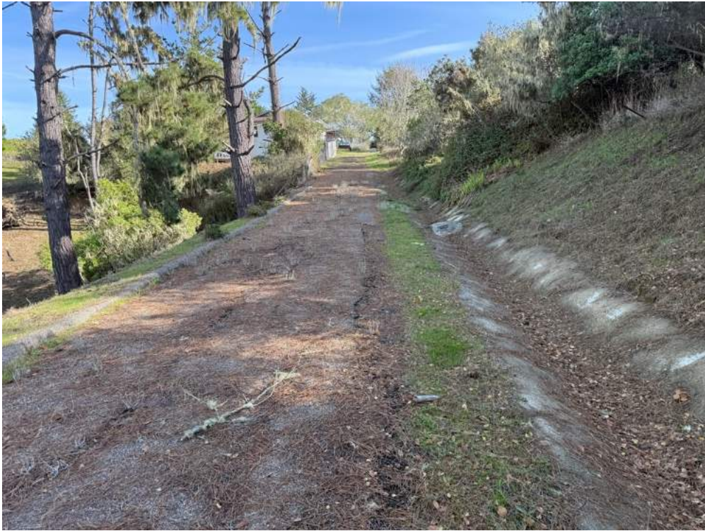
Photo 1. Southeasterly view of an old asphalt road onsite that accesses Skye Street, and a concrete stormwater swale along the road.
