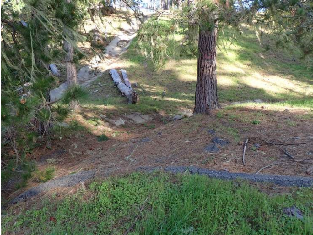
Photo 13. The concrete swales and asphalt curb converge in the eastern part of the bench to direct runoff into a storm drain pipe.
